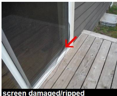
screen damaged/ripped
